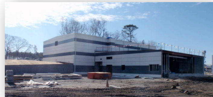
•Hall D (construction)
